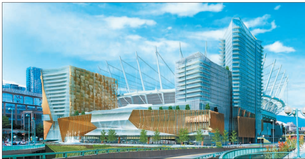
Paragon Gaming Inc. proposes to borrow $350 million and build a $450 million casino adjacent to BC Place
